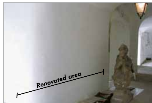
After the restoration with Seccopor
